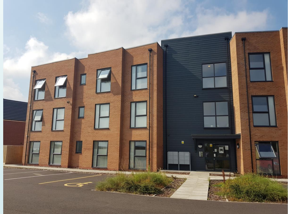
Pic - Beamish Court
